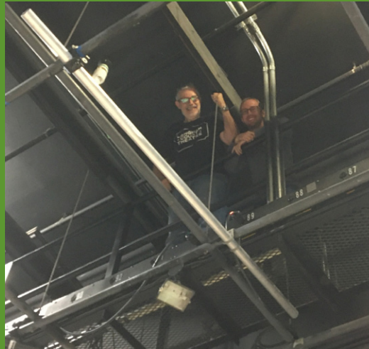
Paul Hilton and Max Terpstra are working in the grid above the stage, getting the lights ready for Rope .
